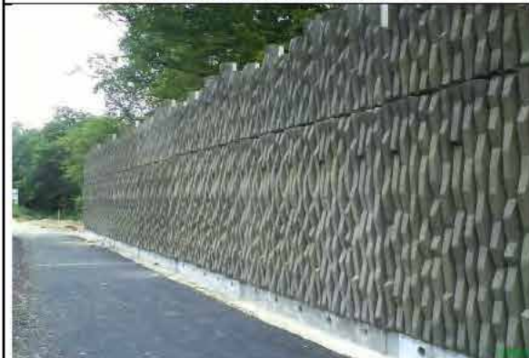
A13, La Celle St Cloud - Le Chesnay - Rocquencourt (78)
